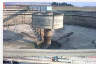
Thabong PST under refurbishment
