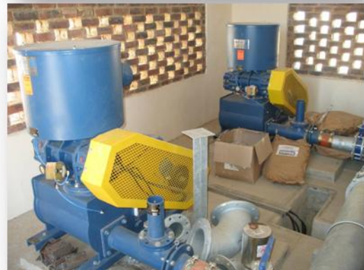
Top: 2008 construction of the new Vredefort plant; Below: new blower motors for diffuse aeration system.
