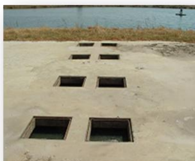
Right: Lindley town pumpstation, screenings removed manually and buried; Left: Primary settling tanks at Lindley plant, with aerated oxidation ponds in background
