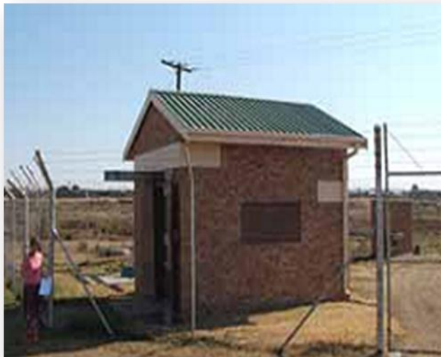
Fenced pumpstation at the Rouxville plant
