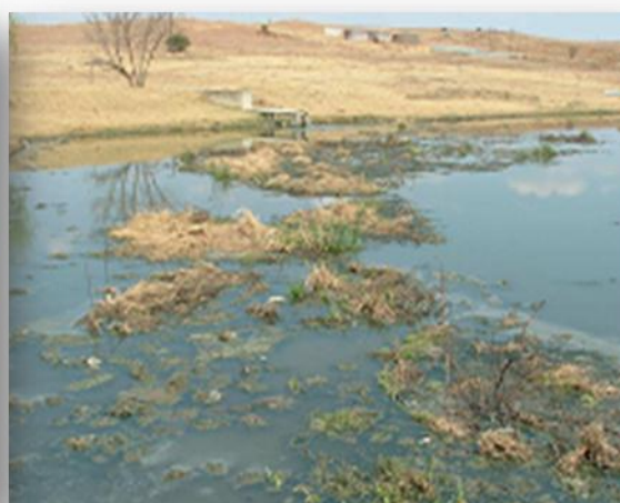
Warden biofilters and pond not functional
