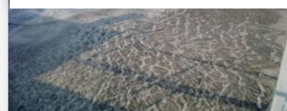
Thabong PST aerators non-functional, build-up of scum in reactor
