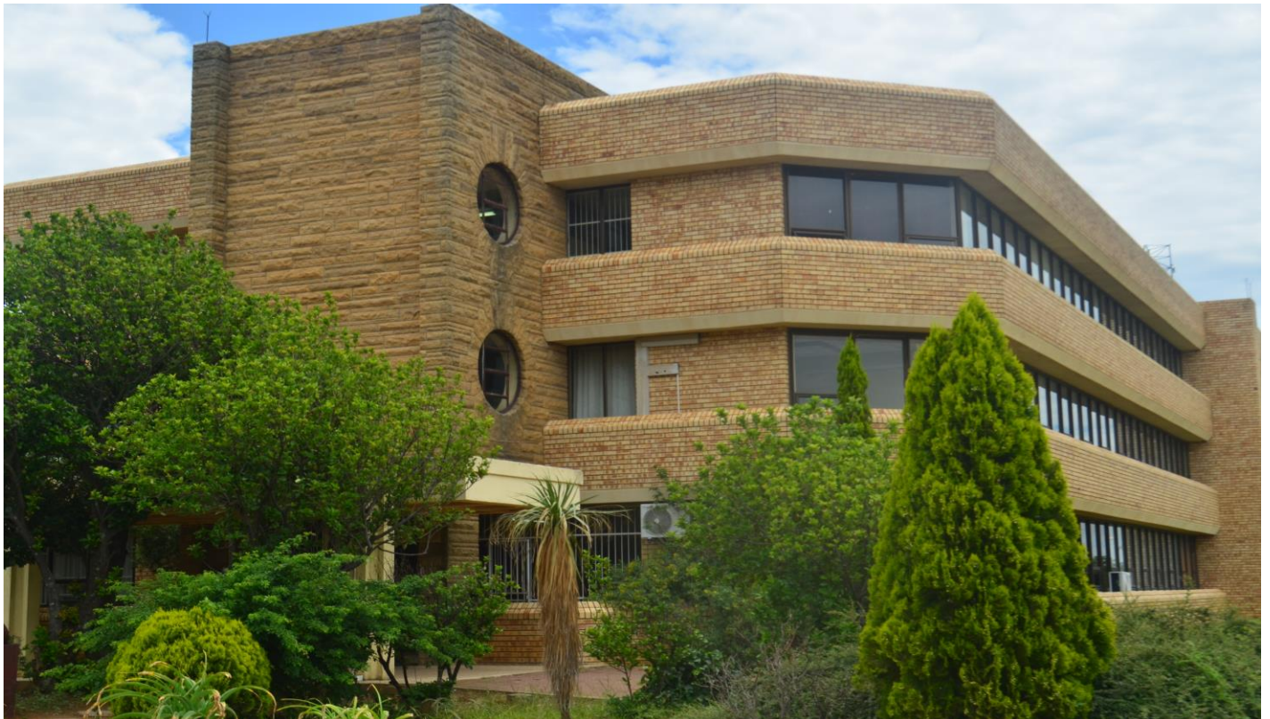
THABO MOFUTSANANYANA DISTRICT MUNICIPALITY OFFICES. OLD PARLIAMENT BUILDING.
